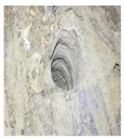
The adhesive-concrete bonding can be detrimentally affected by various conditions including dust or debris left in the drilled hole, temperature and humidity conditions associated with the underlying concrete as well as
